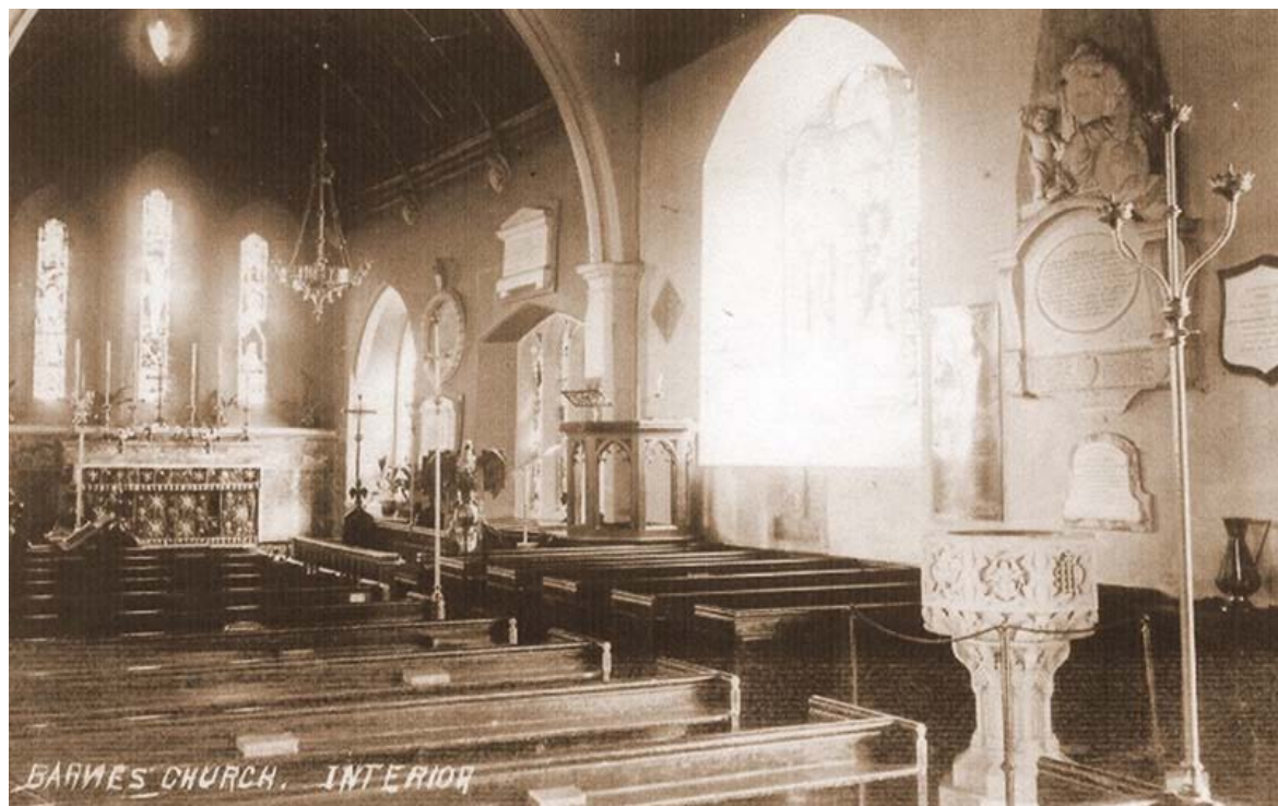
Hoare memorial, c.1788, by John Hickey on the south wall; the site of the 12th century church. Looking east towards the 13th century Langton chapel built as a chancel to the earlier church.
